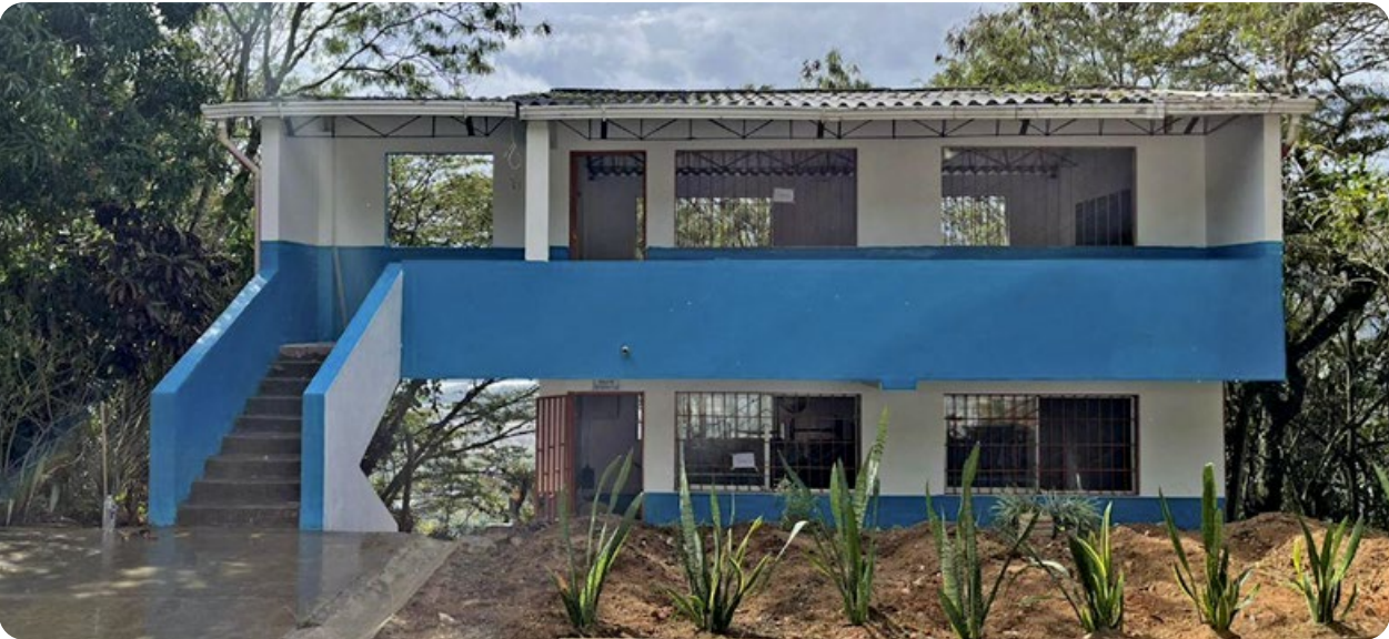
The renovation of La Meseta School’s façade in Girardota, Antioquia, was completed through in-kind donations.
